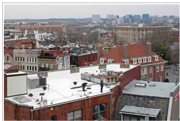
Maria-José Viñas / American Geophysical Union White roofs are being tested around the world, including this one in Washington, D.C.
